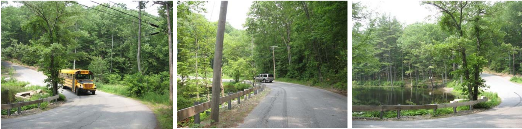
Views showing sharp and blind corner near Heald Pond Dam. Recently installed guard rail was struck by vehicle within its first few weeks of existence.
