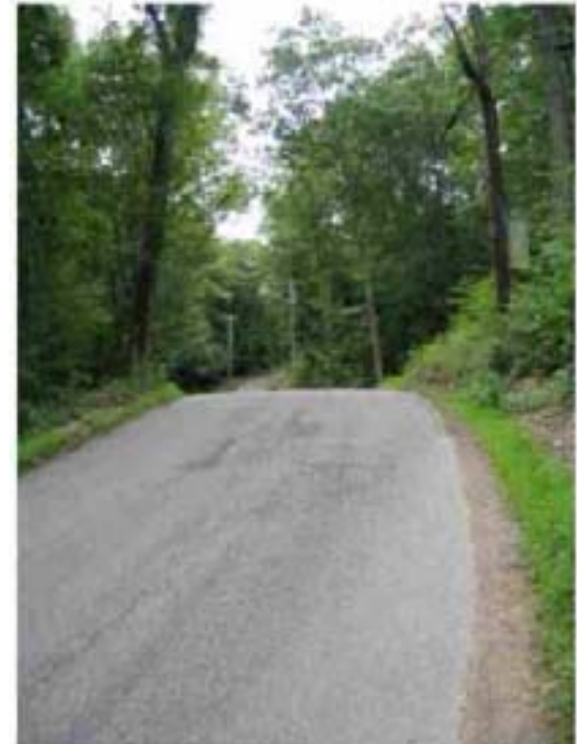
Driver's view when own vehicle's roof becomes visible to driver turning left from Bayberry Rd onto Heald St (You can't even see Bayberry Road Street Sign).
